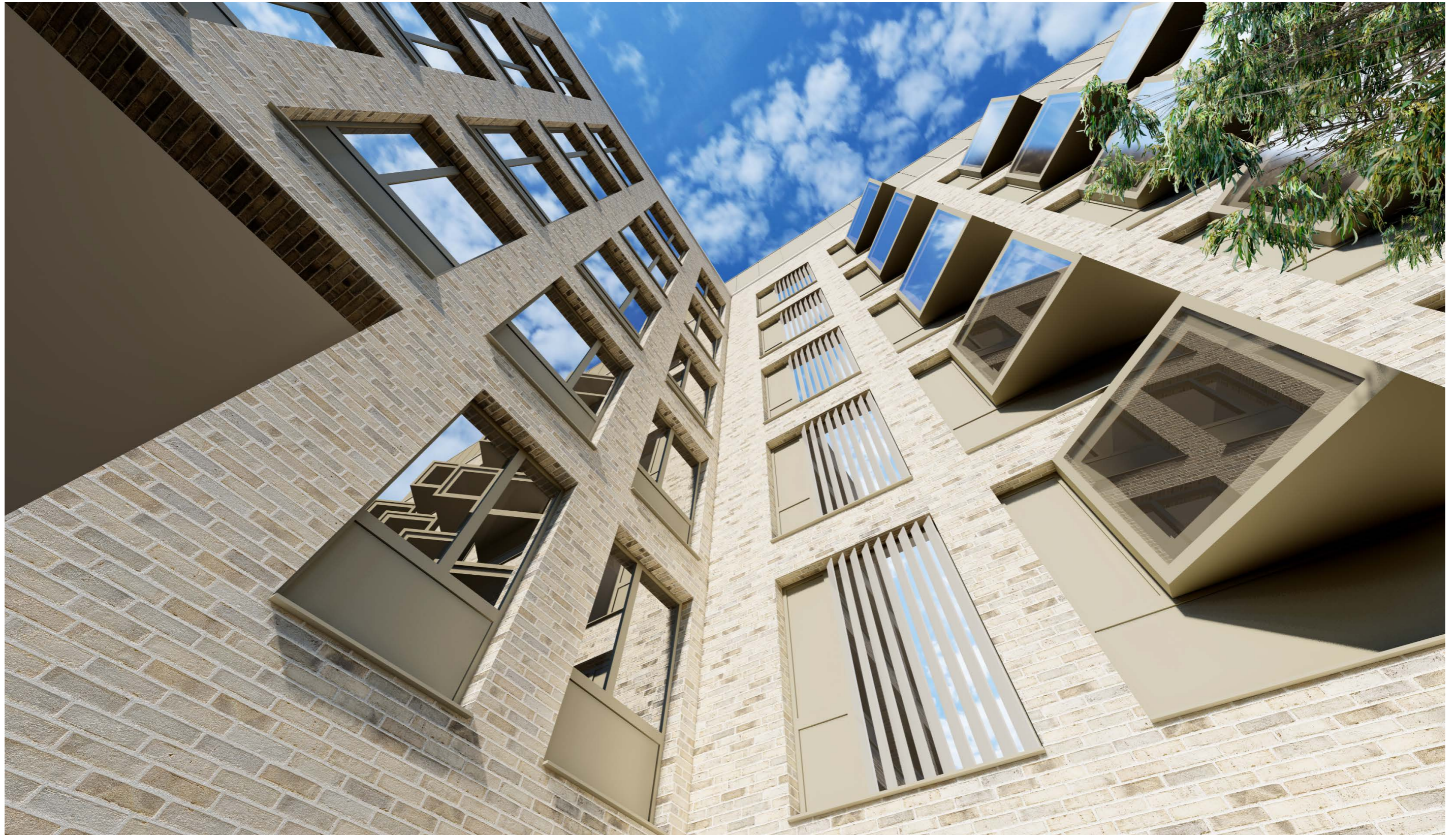
Artists impression - East facade / internal corner inc opaque louvre detail and 'saw-tooth' projecting bay windows
