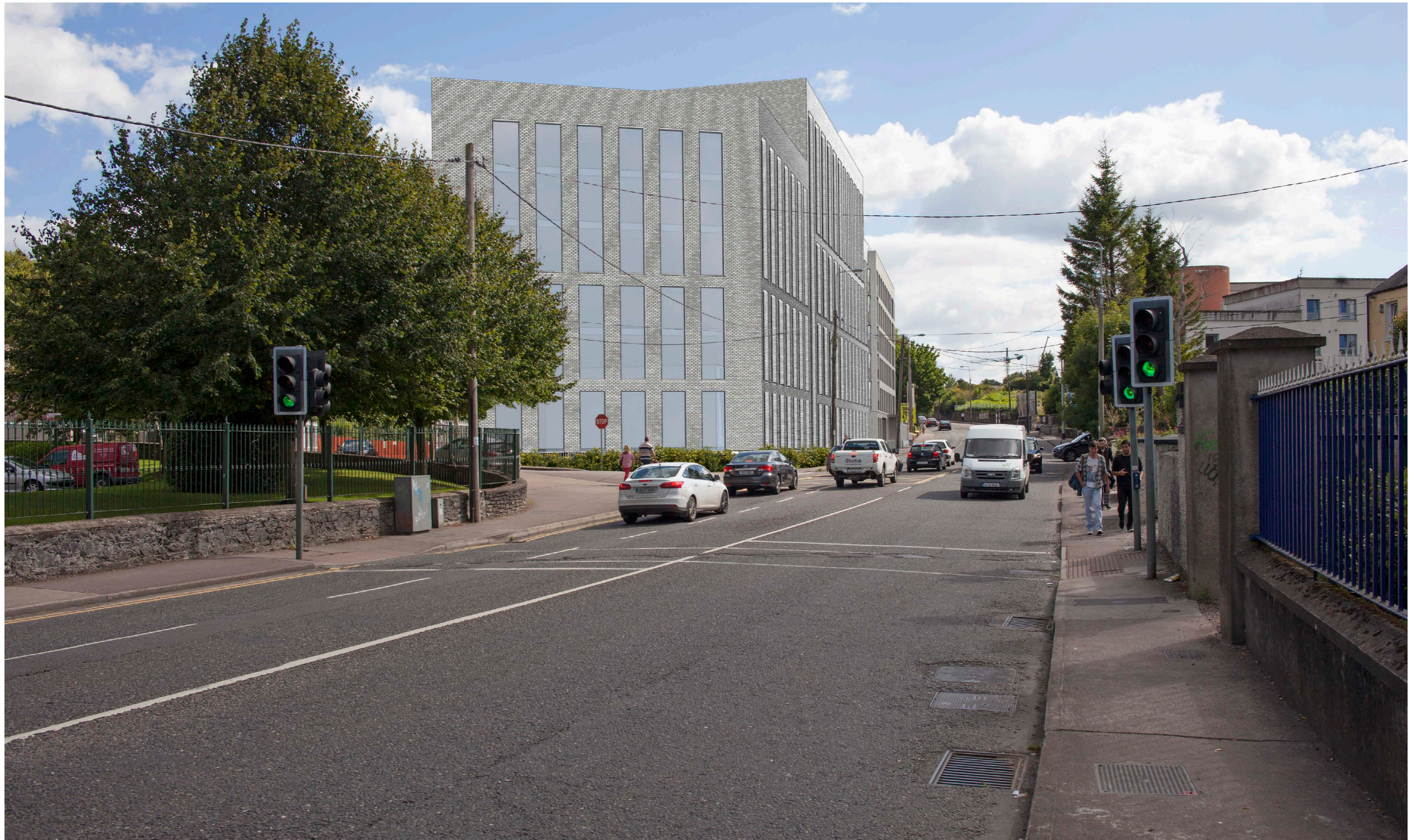
Preplanning LVIA view of preliminary massing with 6-8 storeys to Victoria Cross Road inc as-permitted development (ABP 306714-20)
