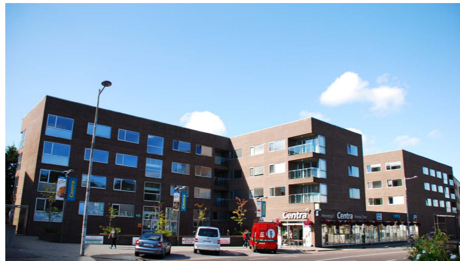
University Hall Student Accommodation, Victoria Cross.
