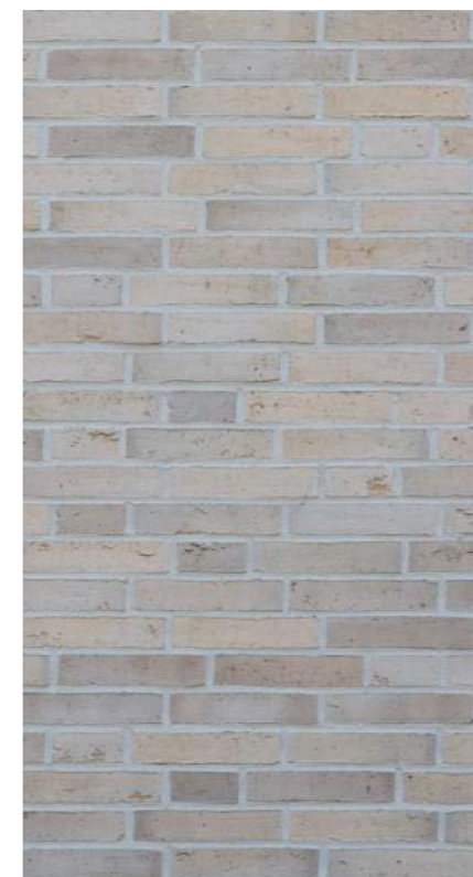
Brickwork Petersen Tegel d190 & Marzial A blend of yellow-grey stock like bricks with white mortar
