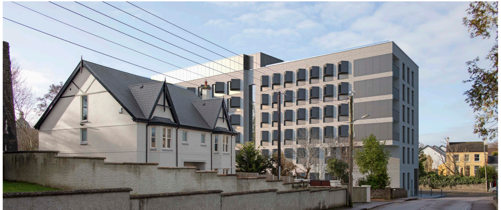
LVIA - East facade 'saw-tooth' projecting bay windows to limit direct overlooking of adjoining properties
