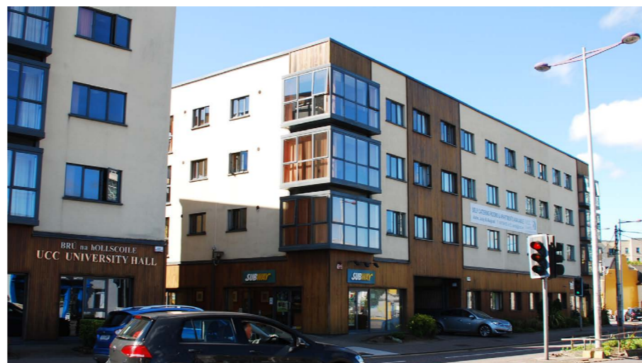
University Hall Student Accommodation, Victoria Cross.
