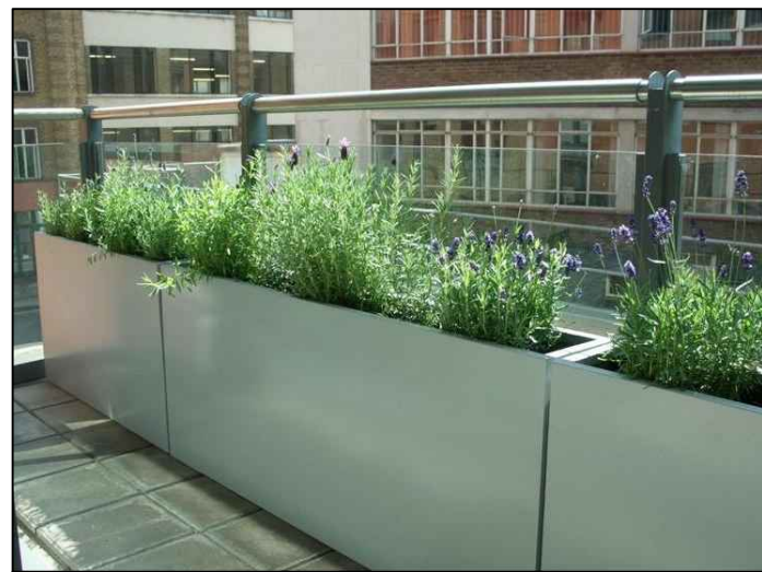
Raised steel planter boundary in front of safety rail
